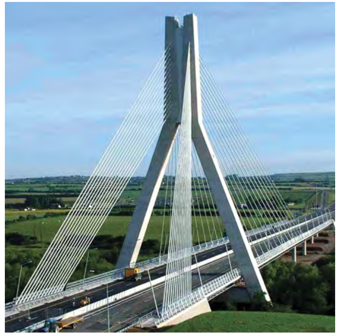
Above: Boyne Bridge M1 motorway Concrete Piers contain GGBS, resulting in a lighter more aesthetic appearance.
