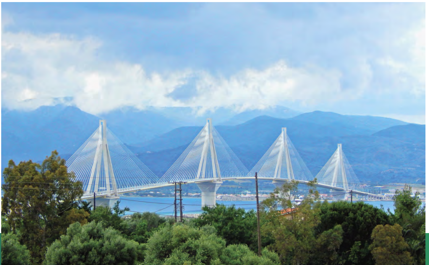
Below: The Rio-Antirion bridge Constructed in 2004 is the world's longest cable-stayed bridge. Its foundations were constructed with a blended cement comprising 60% GGBS for a service life of 120 years. [RCPT values in real life testing were consistently under 300 C]
